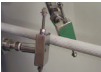
Blowing off water from pipe
